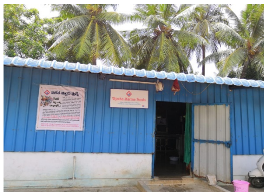
Cold Storage Unit at Bhimavaram
