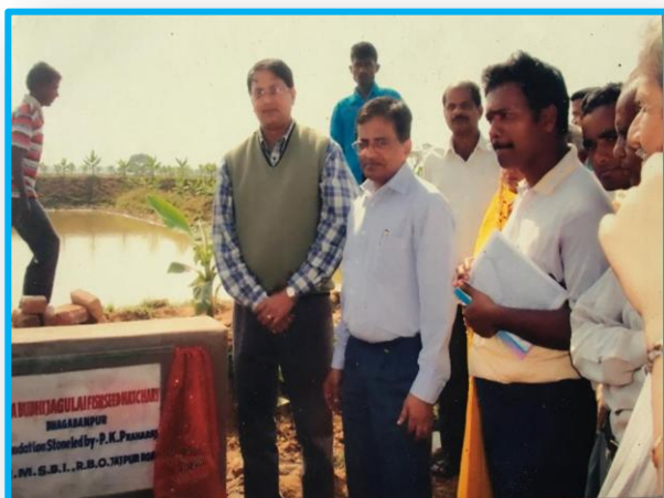
Laying of Foundation stone of Hatchery by Shri P.K. Praharaj, General Manager, SBI in presence of Director, ICAR-CIFA
